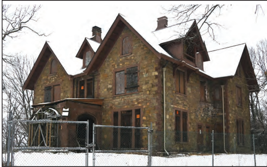
Known as "The Point," the Hoyt house today is stabilized from further deterioration while it awaits restoration and a new purpose for its historic spaces.
