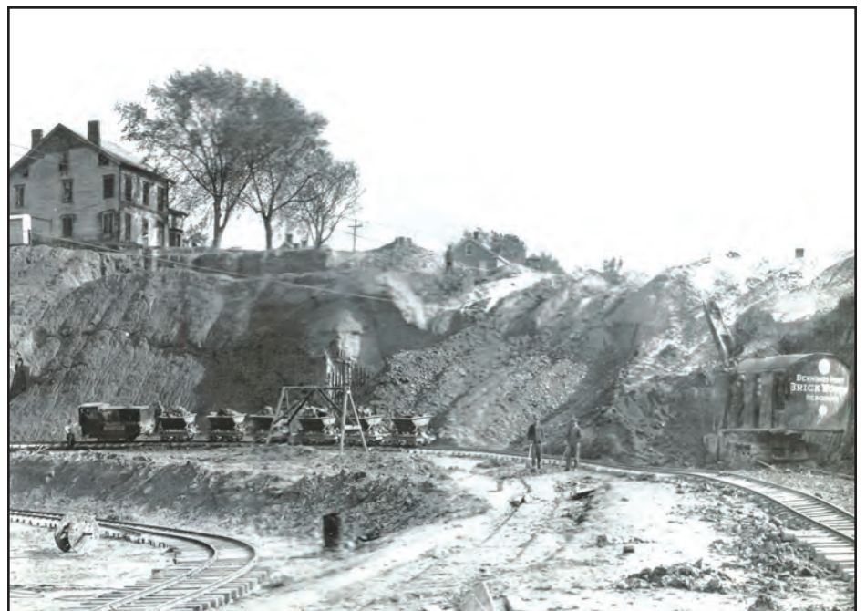
The introduction of an electric train and shovel dramatically improved the efficiency of the Denning's Point Brickyard in 1926.
