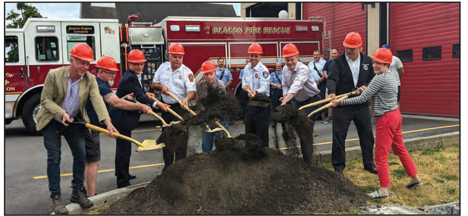
A symbolic groundbreaking took place for the renovation and addition of the City of Beacon’s new consolidated firehouse, which is the Lewis Tompkins Hose fire station. Pictured (left to right): City Councilmember-at-Large George Mansfield; Assistant Volunteer Fire Chief Dennis Lahey Jr.; City Administrator Chris White; Former Beacon Fire Chief Gary VanVoorhis; Former Volunteer Fire Chief Dennis Lahey Sr.; Beacon Fire Chief Thomas Lucchesi; Ward Four City Councilmember Dan Aymar-Blair; Mayor Lee Kyriacou and Ward One Councilmember Molly Rhodes.
