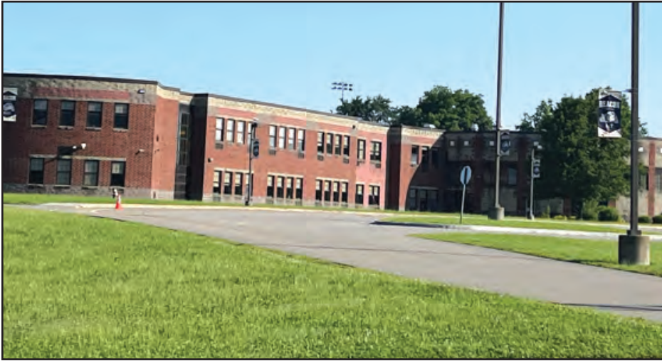
In a recent update to the community, Beacon City School District Superintendent Dr. Matthew Landahl wrote about the upgrades to the HVAC system at Beacon High School, which are set to begin over the summer.
