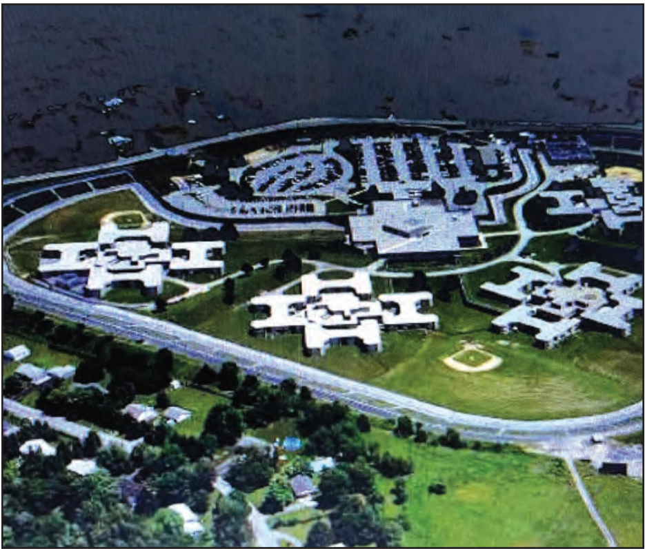
New York State is seeking proposals for the former Downstate Correctional Facility. The site has been decommissioned.
