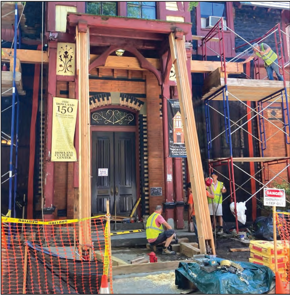
Renovation work continues on the Howland Cultural Center, on Main St., in Beacon.
