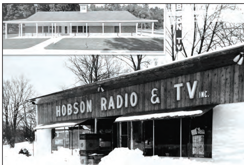
Bottom: The building at 6282 Route 9, Rhinebeck, known for over half a century as Hobson's Radio & TV, has been carefully crafted for site-sensitive adaptive reuse as the headquarters of the Dutchess County Historical Society's libraries and archive.
