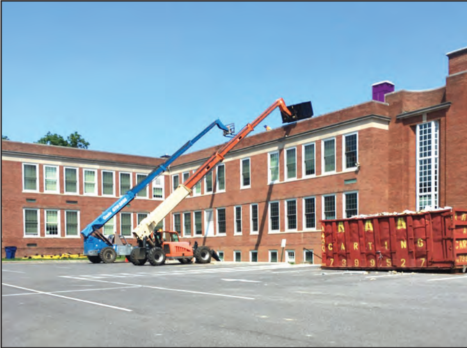
The roof demolition at Wappingers Junior High School during the summer.
