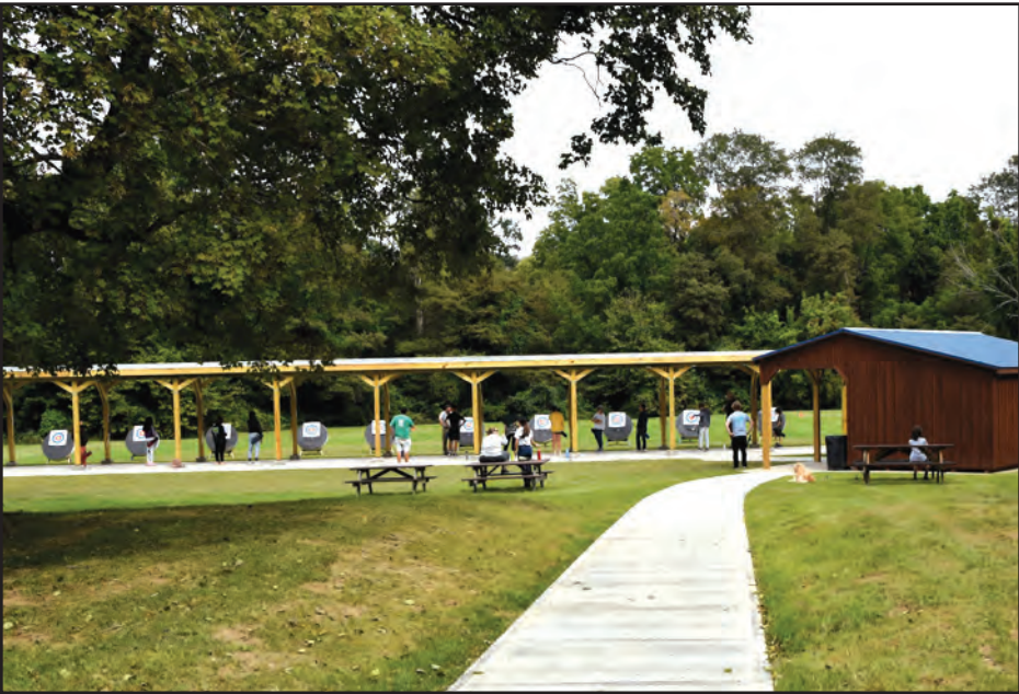
The new archery range at Bowdoin Park was completed this summer with funds received through the federal American Rescue Plan (ARP) Fund and expands capacity for the popular program held every spring and fall as part of Parks’ Naturalist Programming schedule.
