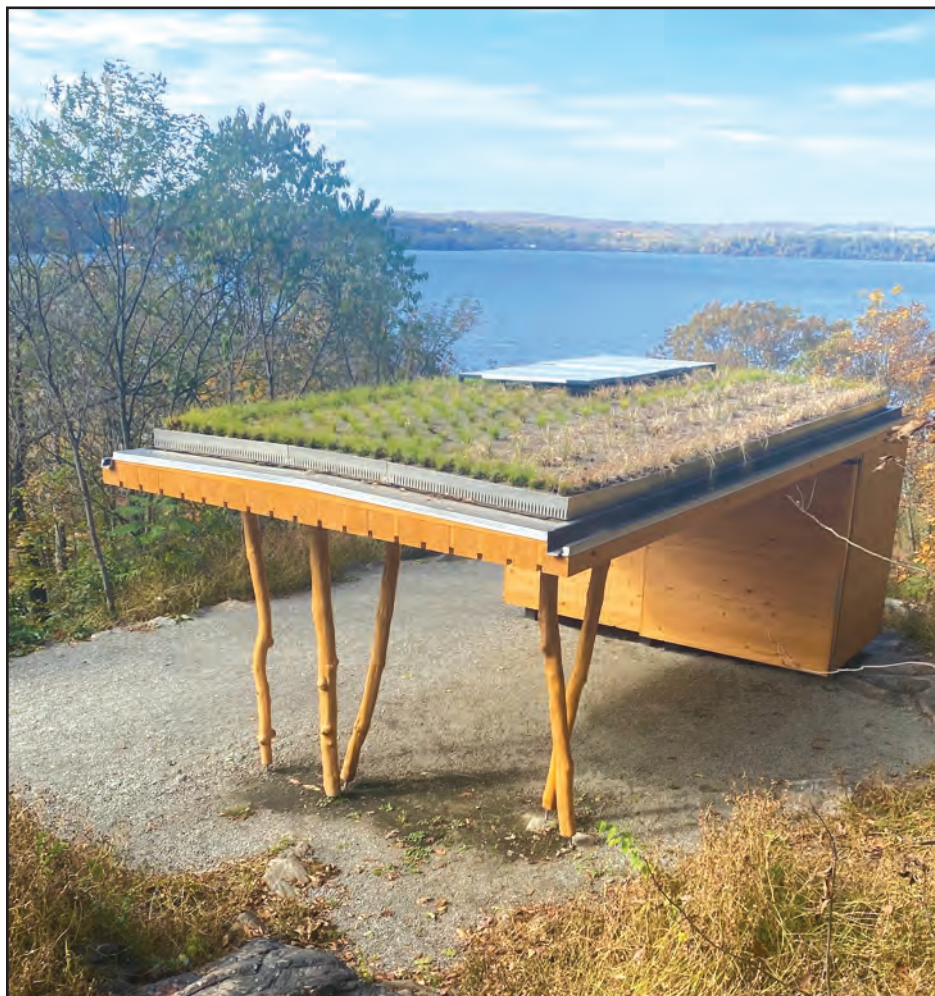
Trail Steward Station solar panels.
