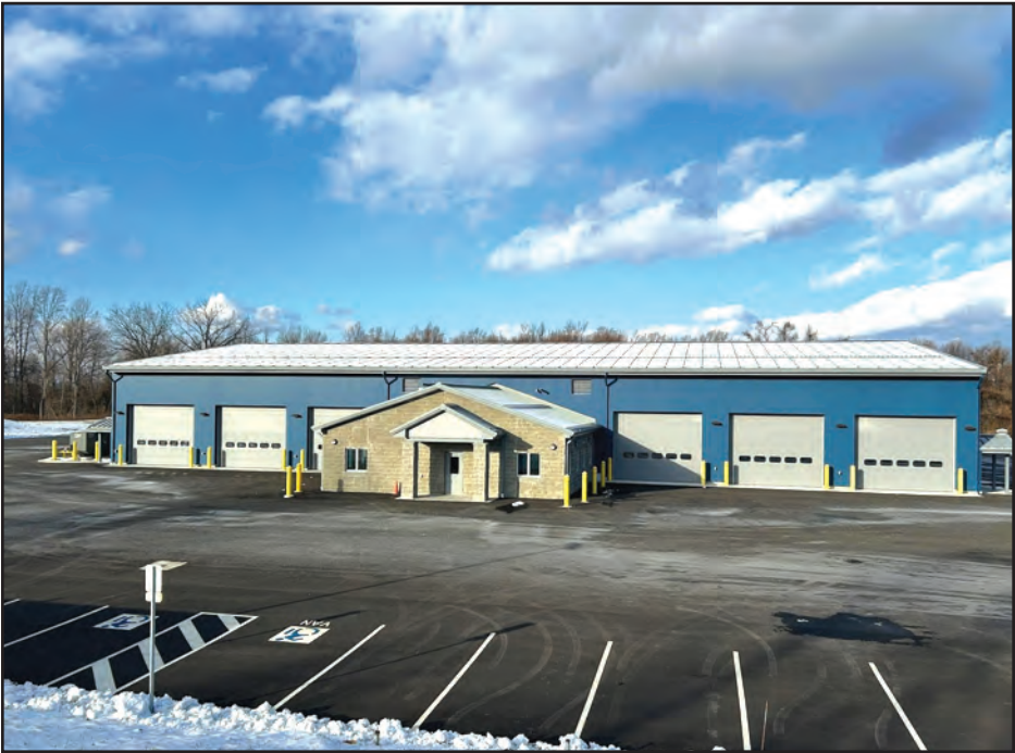
The new NYS DOT maintenance facility in East Fishkill.
