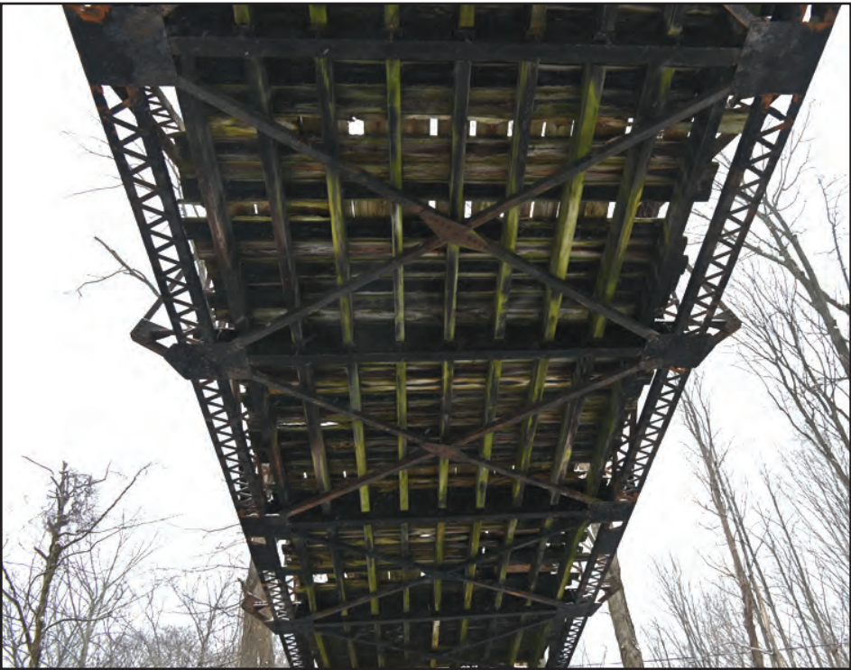
The underside of the Hoyt Carriageway Bridge's wooden deck is shown above. There is a lot of light coming through and it is no longer safe. The restoration plan will have the wood of the deck replaced this spring so that the bridge can support pedestrian traffic in time for the summer hiking season.
