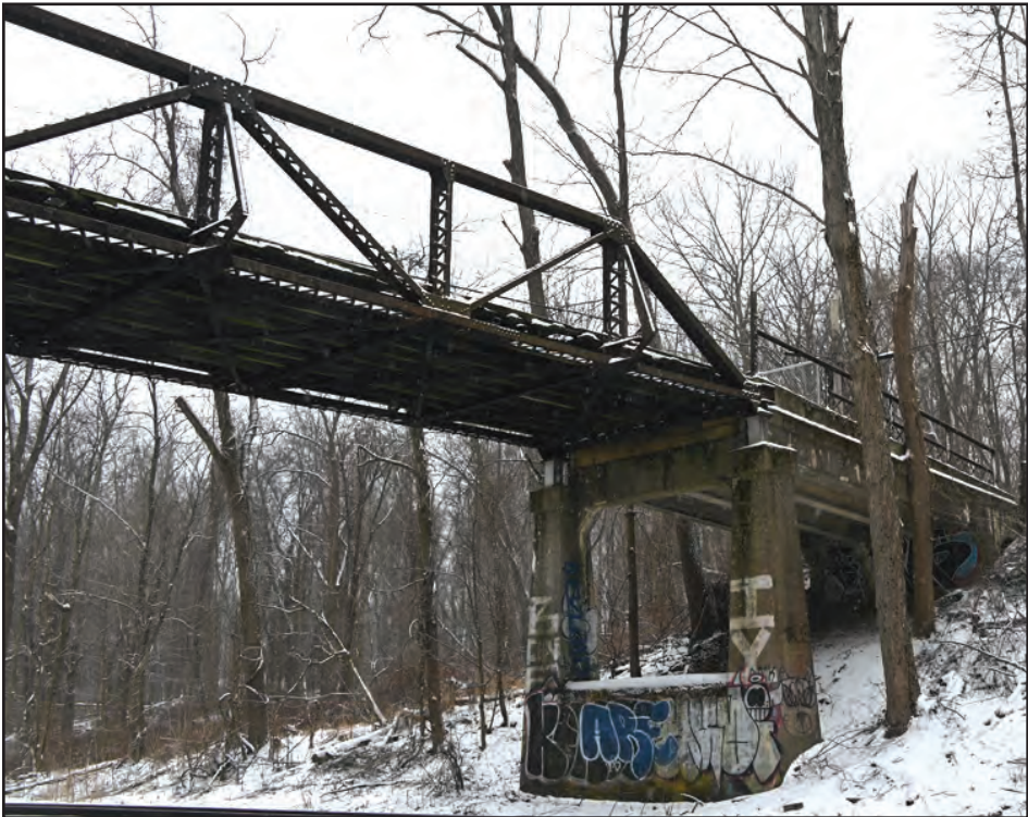
After years of neglect, the 112-year-old Hoyt Carriageway Bridge looks to be ready for a good cleanup and restoration. Even after so many years, the basic structure is sound and the majority of the restoration effort will be replacing the lumber on the wooden deck, then sand-blasting and painting. There is even hope that removal of so many years' graffiti may encourage local artists to find a different canvas for their work. Below: Known as "The Point," the Hoyt house today is stabilized from further deterioration while it awaits restoration and a new purpose for its historic spaces. All photos by Jim Donick
