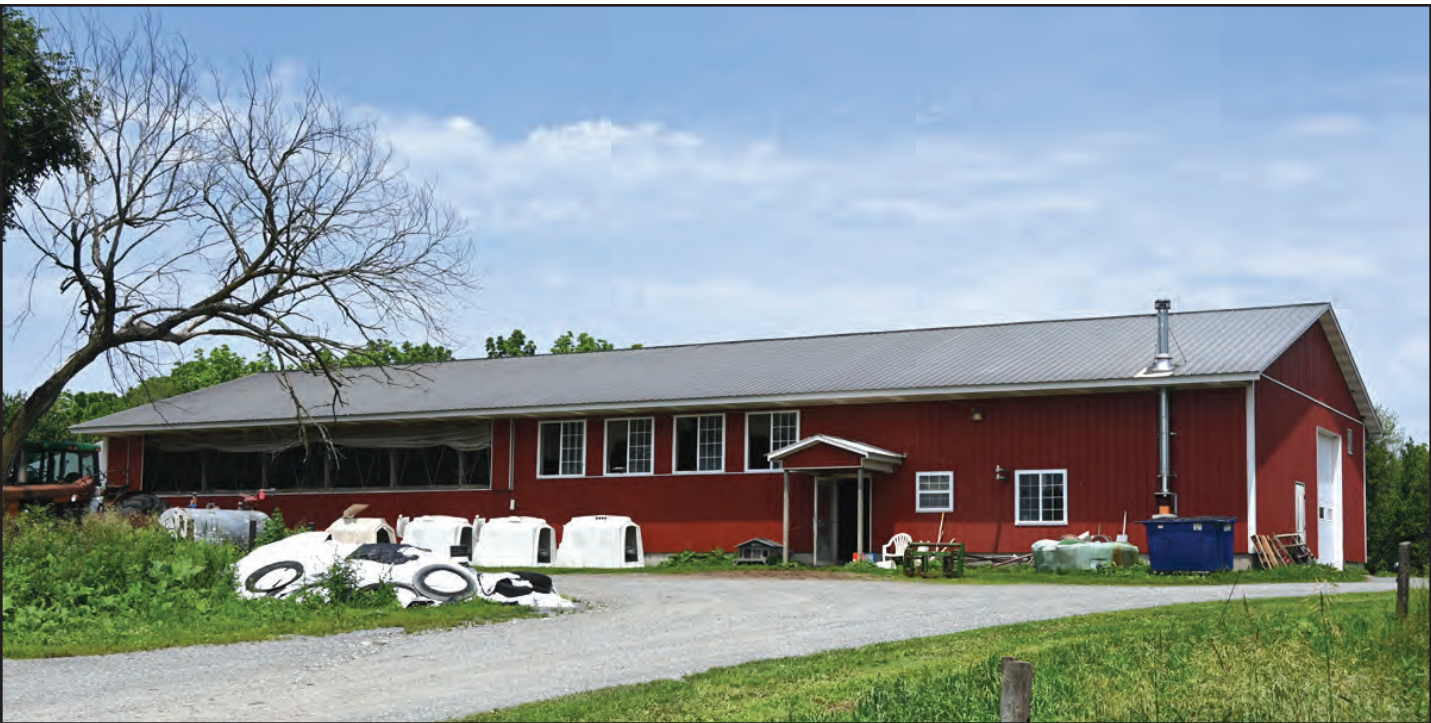
The new barn at Uplands Farm in Verbank will house the new 3,000-gallon holding tank for milk. Photo by Jim Donick
