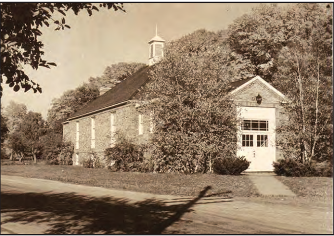
Rhinebeck Grange #896 was established on November 12, 1900. Pictured above is the Rhinebeck Grange Hall (now a law office). Courtesy photo
