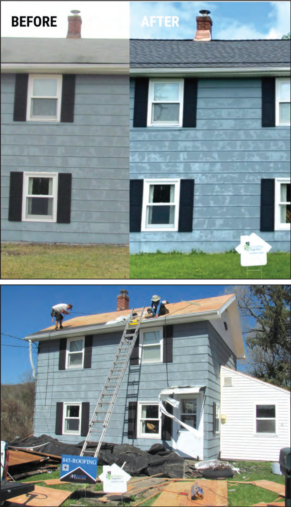
From top: Before and after photos of the Amenia roof replacement project. The project in process by Rebuilding Together Dutchess County. Courtesy photos
