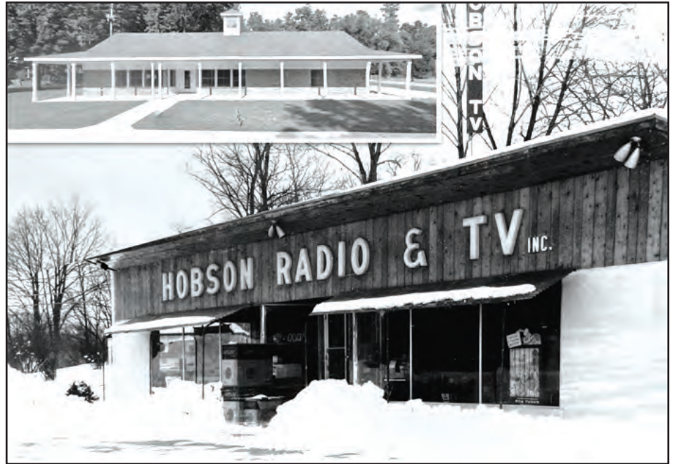
The building at 6282 Route 9, Rhinebeck, known for over half a century as Hobson's Radio & TV, has been carefully crafted for site-sensitive adaptive reuse as the headquarters of the Dutchess County Historical Society's libraries and archive. Courtesy photos
