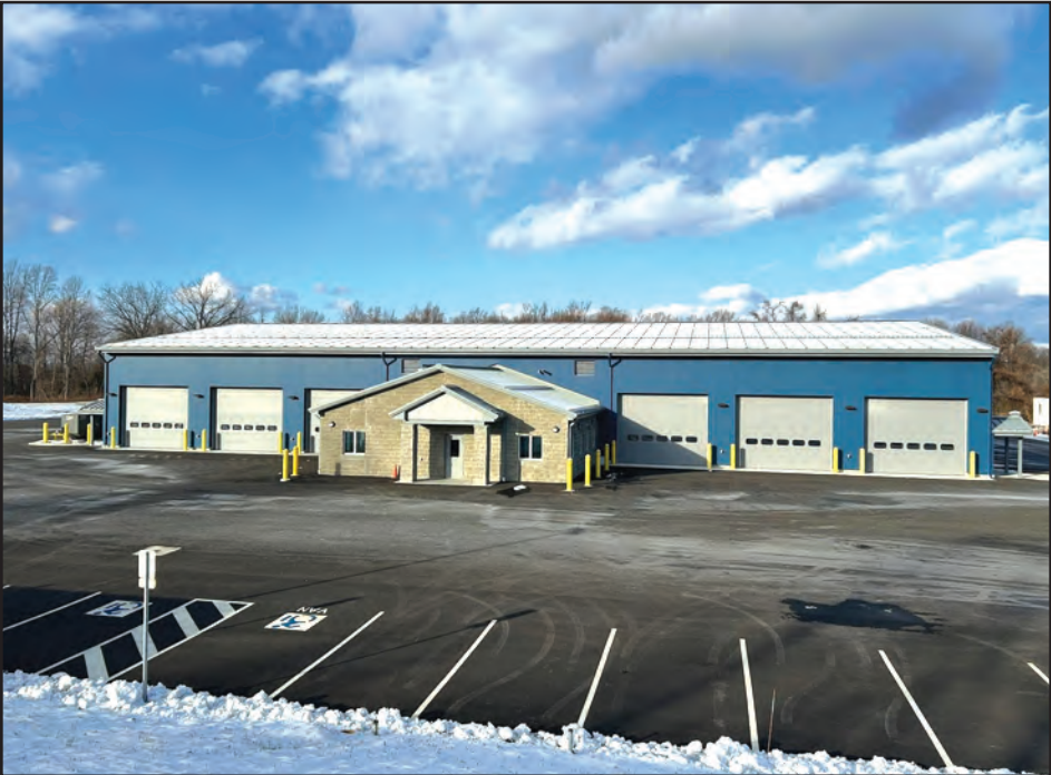
NYS DOT's new state-of-the-art maintenance facility in East Fishkill. Courtesy photo
