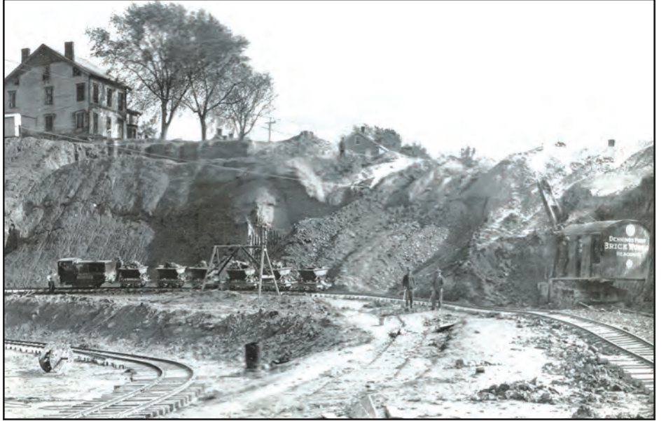
The introduction of an electric train and shovel dramatically improved the efficiency of the Dennings Point Brickyard in 1926.
