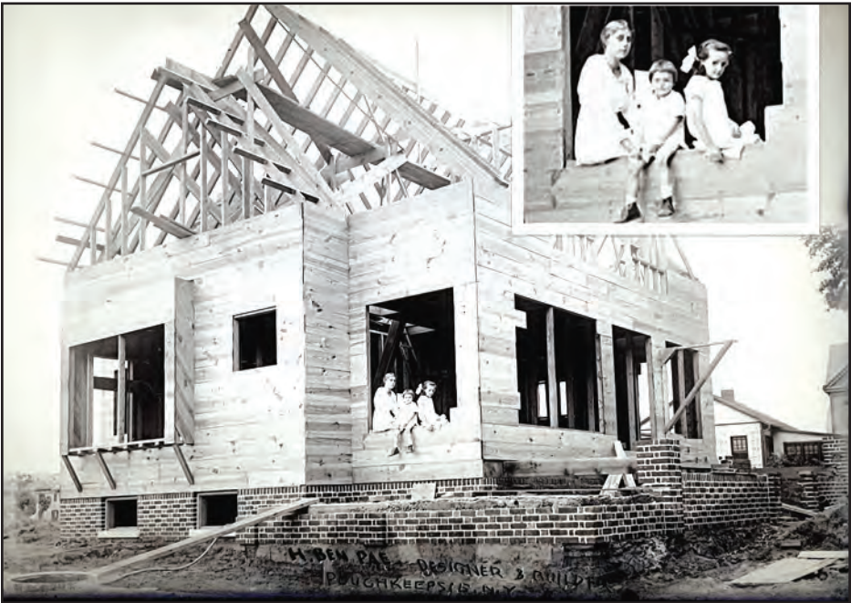
These photos from glass plate negatives show construction of a more permanent home we believe was near the factory of the New York Portable Bungalow Company near today’s Marist University. Ben Pae’s wife, Elizabeth, died in February of 1914 when daughter Marion was five years old, and son Wilfred was only one. We believe this photograph is ca. 1917 showing his children with the woman he married in 1921, Josephine Masten.
