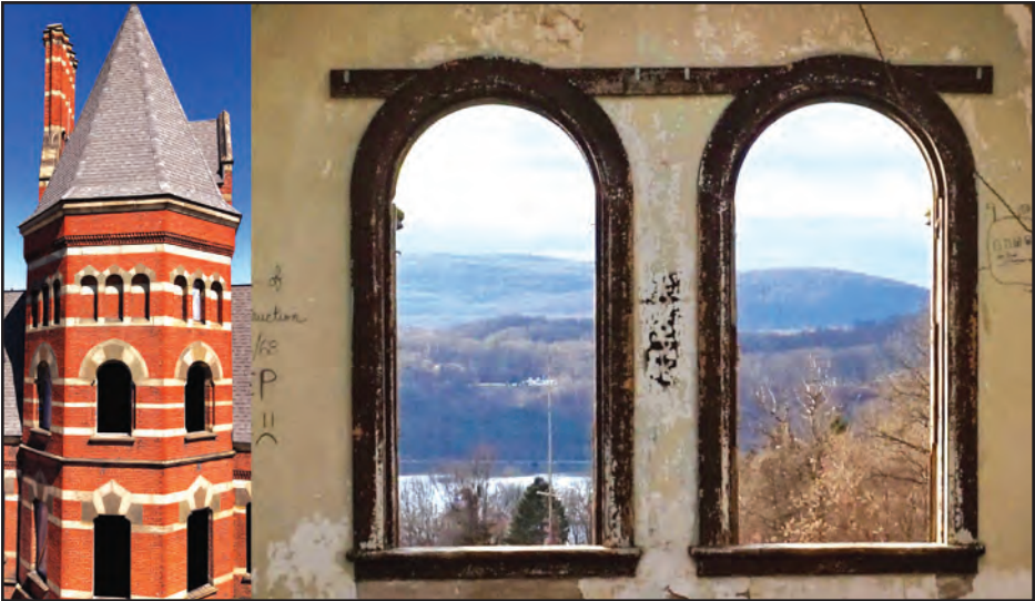
Above left: The architect Frederick Withers brought building materials from Ohio, the Susquehanna and more locally from Croton and the Catskills, to create a spirited, polychrome far-reaching facade. Architectural features inside were designed to be in the supporting role of drawing and framing the view of the outside. -DCHS Image Collection.
