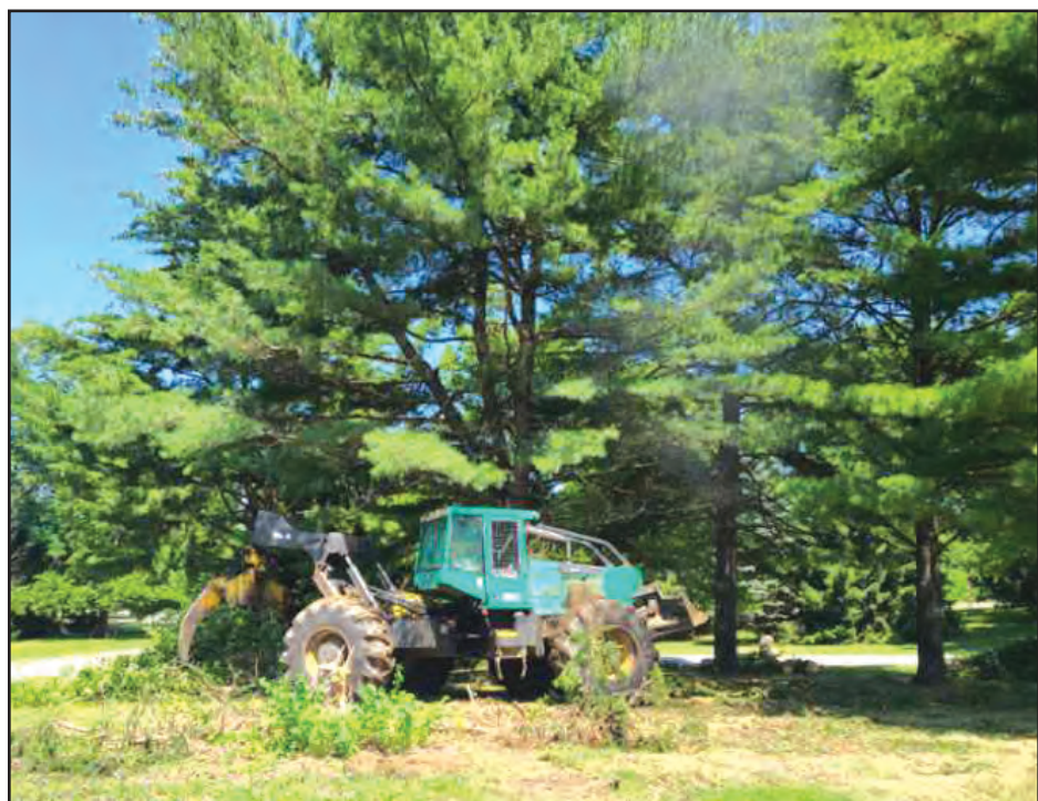
Part of the tree removal/parking lot expansion at Myers Corners Elementary School.
