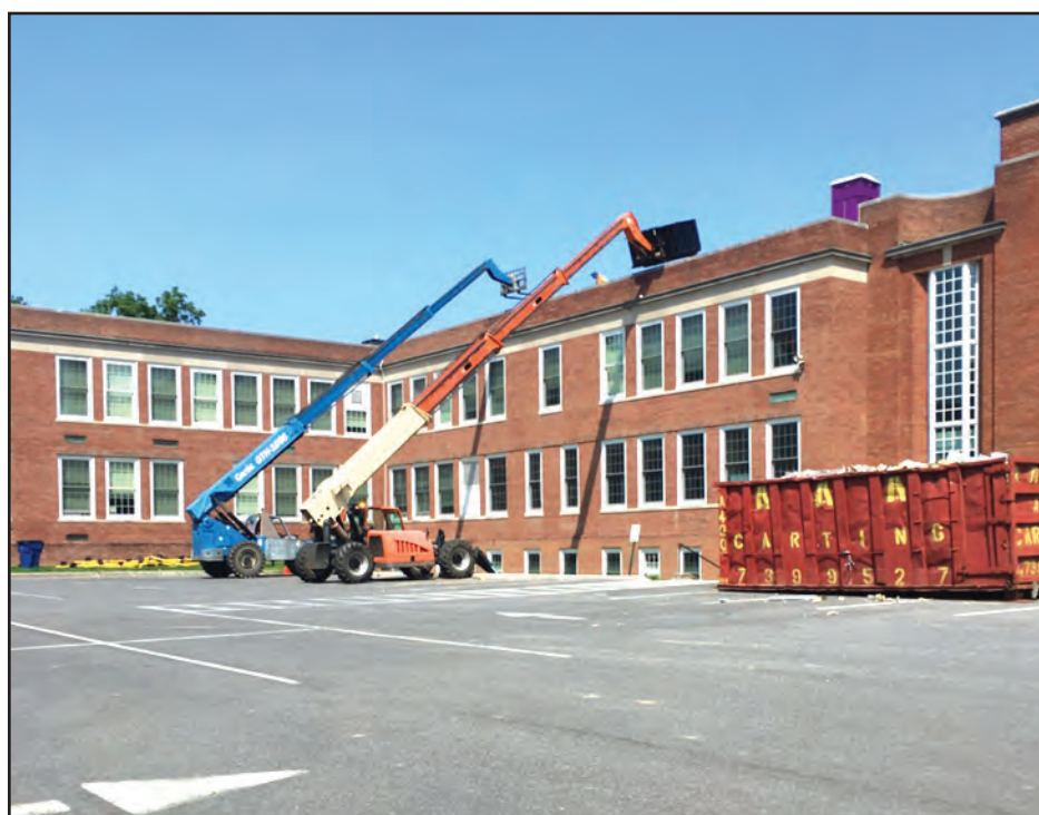
The roof demolition at Wappingers Junior High School during the summer.
