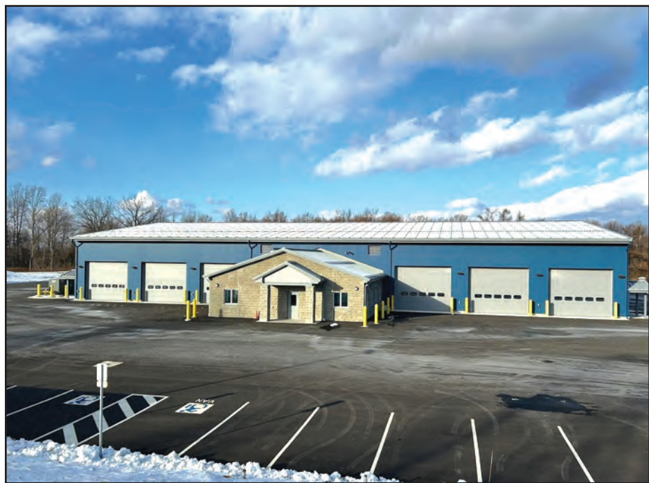
The NYS DOT maintenance facility in East Fishkill.
